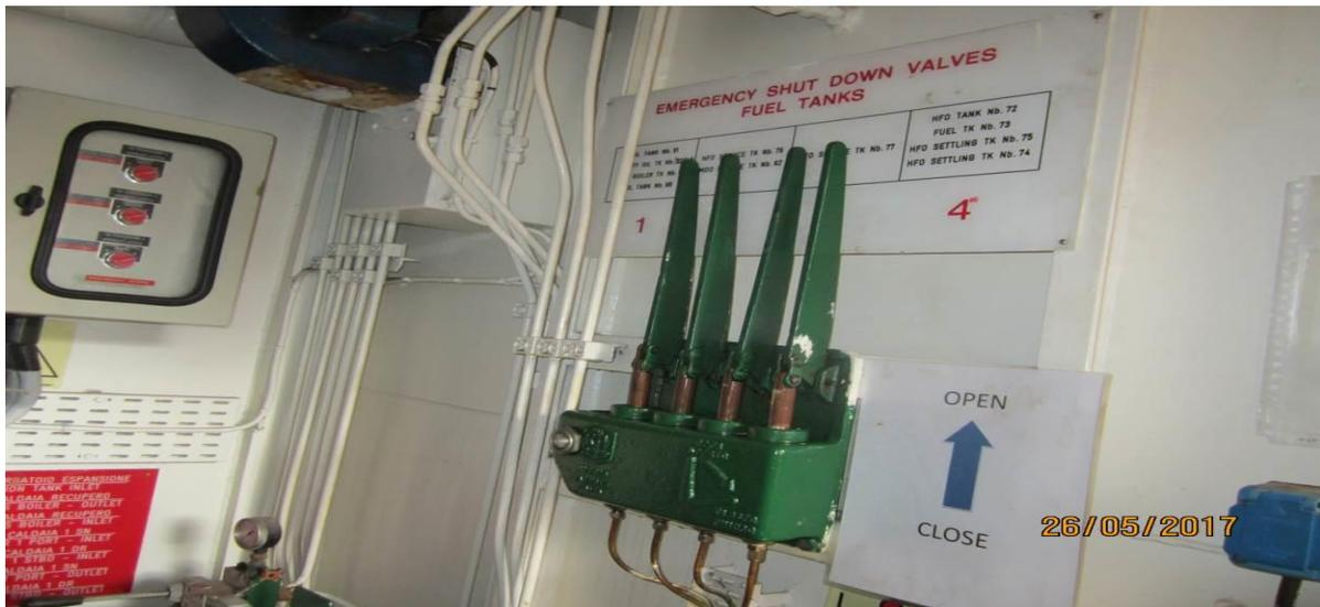
Fig.4 Operating levers for Fuel System Quick Closing Valves (QCV)
