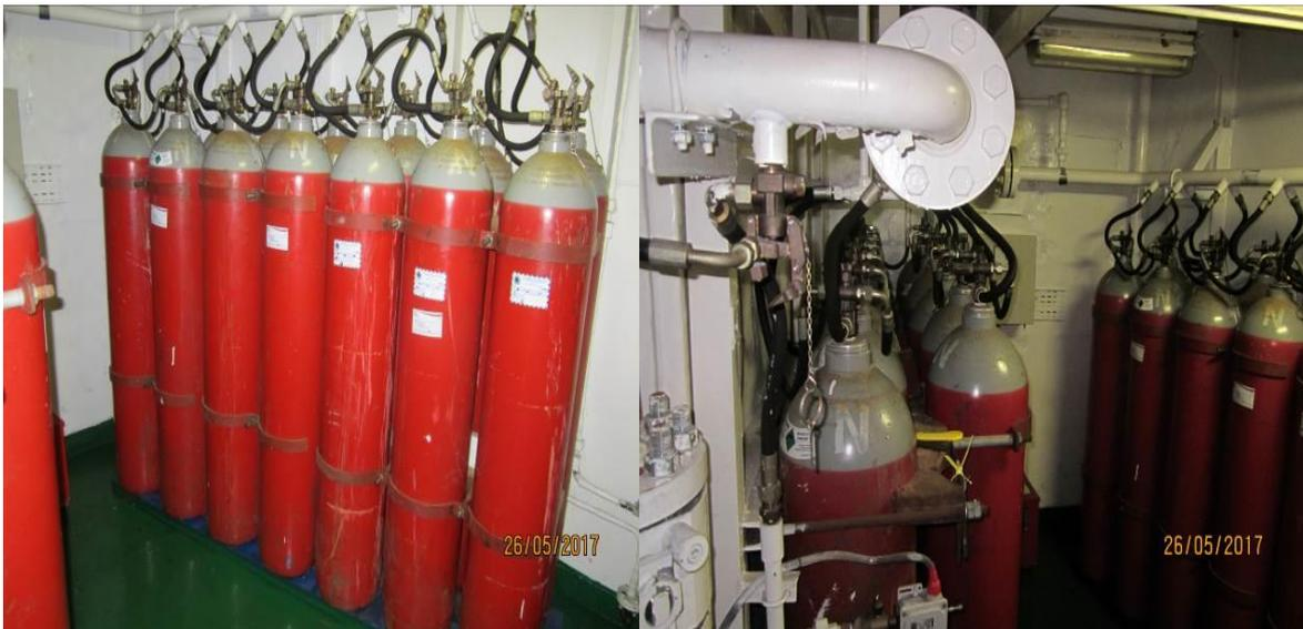
Fig.8 General view of CO<sub>2</sub> station
