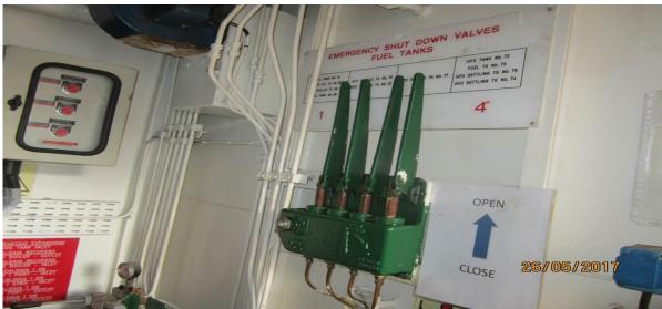
Fig.4 Operating levers for Fuel System Quick Closing Valves (QCV)
