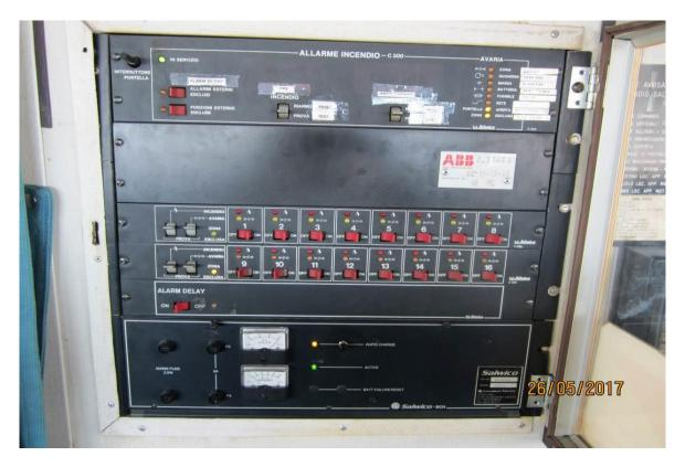
Fig.6 Fire detection alarm panel on the bridge
